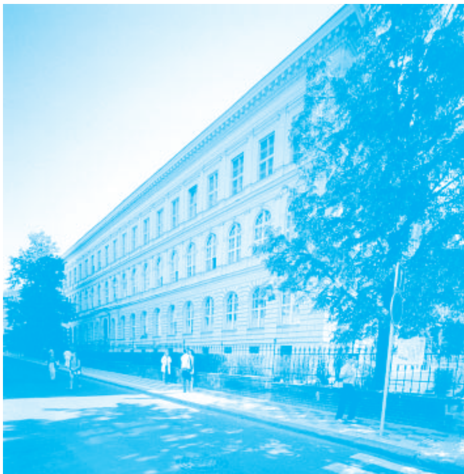
The building of the Dean's Office of the First Faculty of Medicine in 32 Kateřinská, Prague 2.
